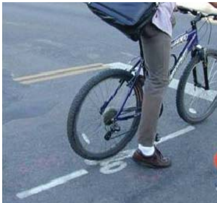
Bike detector markings can be placed at intersections to tell riders where to line up to trigger the signal detectors.
